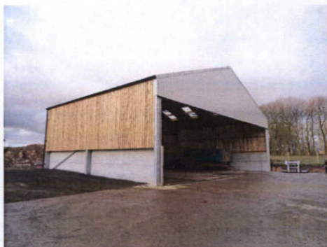
Manure storage building
