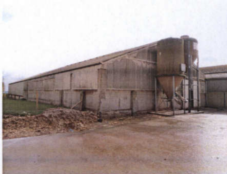
Existing pig building
